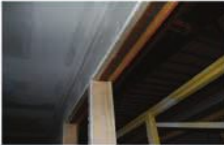
Steel Ceiling Rim w/ LVL at Mateline
