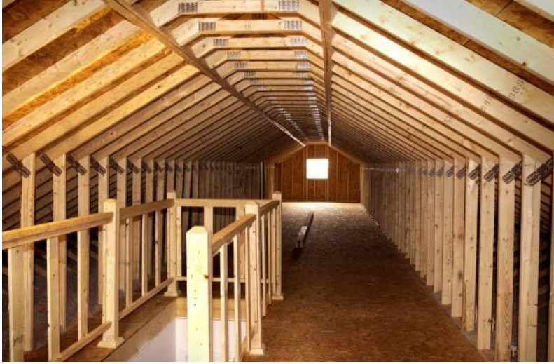
Walk-Up Attic - Shown with optional Attic Window. Available only with 6.98/12 Roof Pitch. Attic Railing built on-site by others and Ridge Beam size shown here varies per model and may protrude up in Attic Space.
