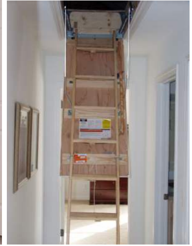
Attic Access with Pull Down Stairs
