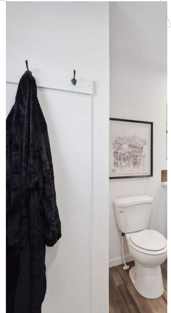
WATER HEATER ACCESS WITH COAT HOOKS
