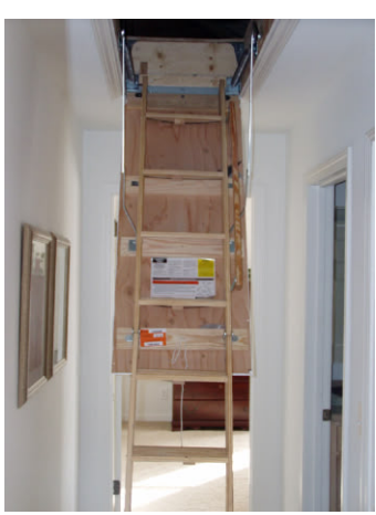
Attic Access with Pull Down Stairs
